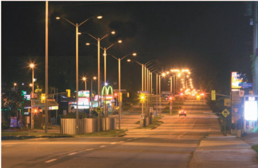
Figure 7 Re-lamping a major street. The benefits of FCO luminaires over semi cut-off fixtures are evident. However, roadside commercial signage should be addressed. After-hour signage for closed businesses should be turned off. Minimal traffic does not require 'rush hour' light levels. (Photo by the author)
