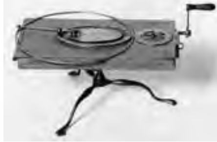
Figure 1 – Cometarium designed by John Rix, ca. 1750. Photograph courtesy of the Smithsonian Museum.
