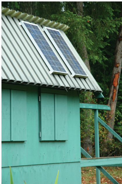
Figure 1 — The roof was built to accommodate the panels. They would need a support frame to get the right angle anywhere else.
