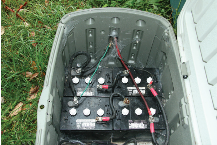
Figure 4 — The batteries live in a Rubbermaid-type garden storage box with vents cut in the ends. Lots of other things live there too. Vents are needed because lead-acid batteries produce hydrogen that is extremely corrosive and even more explosive.
