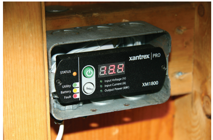
Figure 3 — The remote switch is located beside the door. The readout can show input voltage or current drawn from the batteries.
