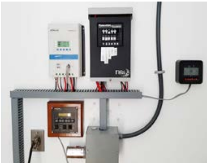
40A MPPT Battery Charging System, Fuse Panel, Power Meter & Lightning Arrestor
