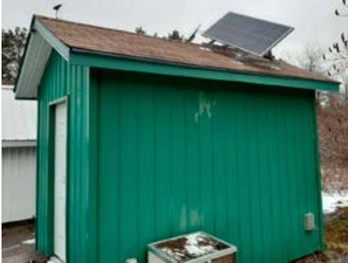
Figure 1: Solar Panels on Roof of Fingal Warm-up Room
