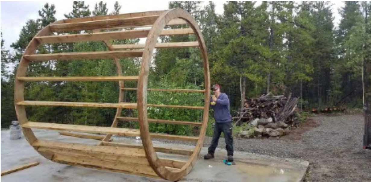
Frame of the new observatory wall
