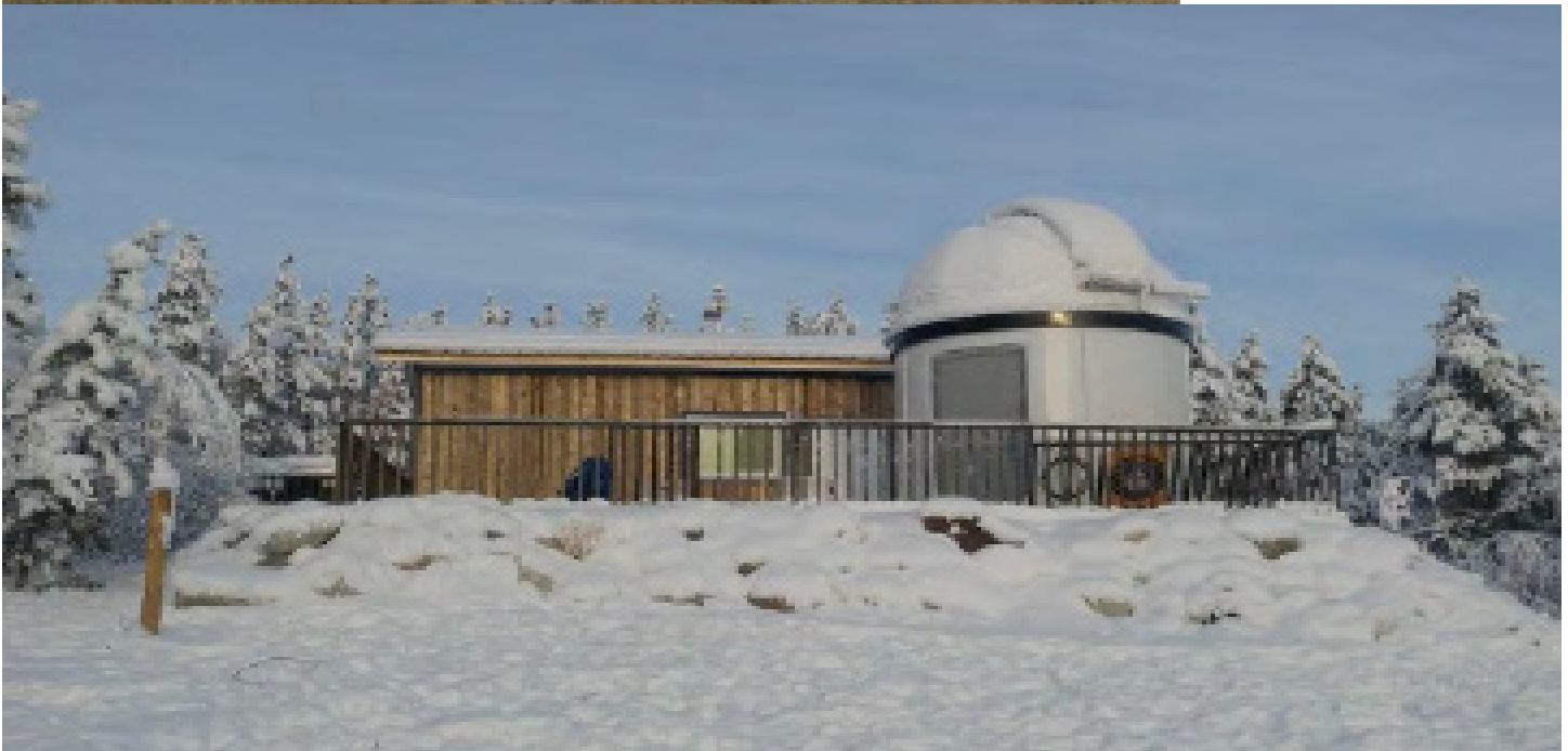
Below: AND...as of completion in February 2019
