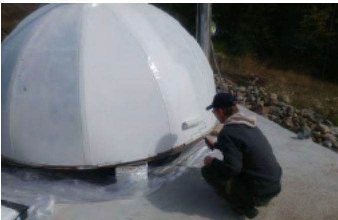
YAS volunteers contributing to construction
