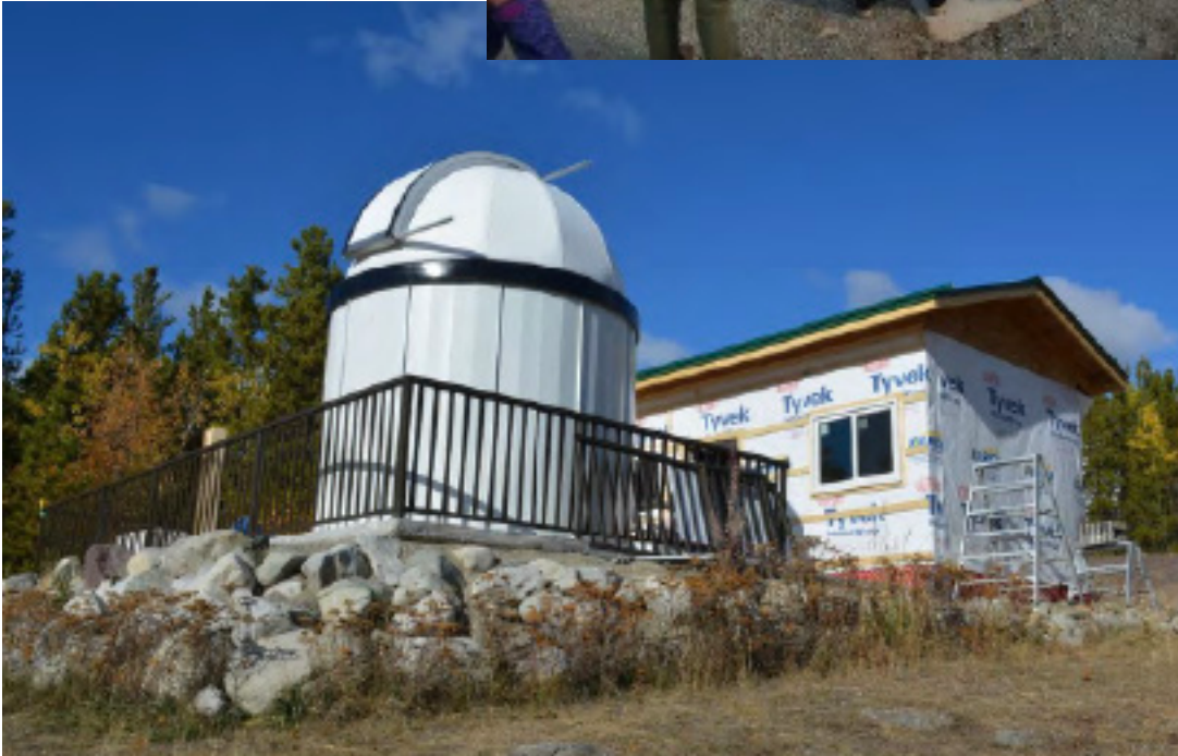
Left: With construction of our Education Centre in progress (September/October 2018) (Courtesy: Chrisv Gainor)
