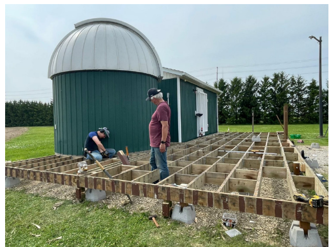
Hallam Observatory deck construction ~ May 2025. Photo by Grant Maguire
