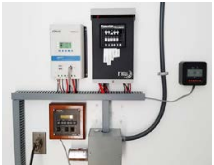
40A MPPT Battery Charging System, Fuse Panel, Power Meter & Lightning Arrester
