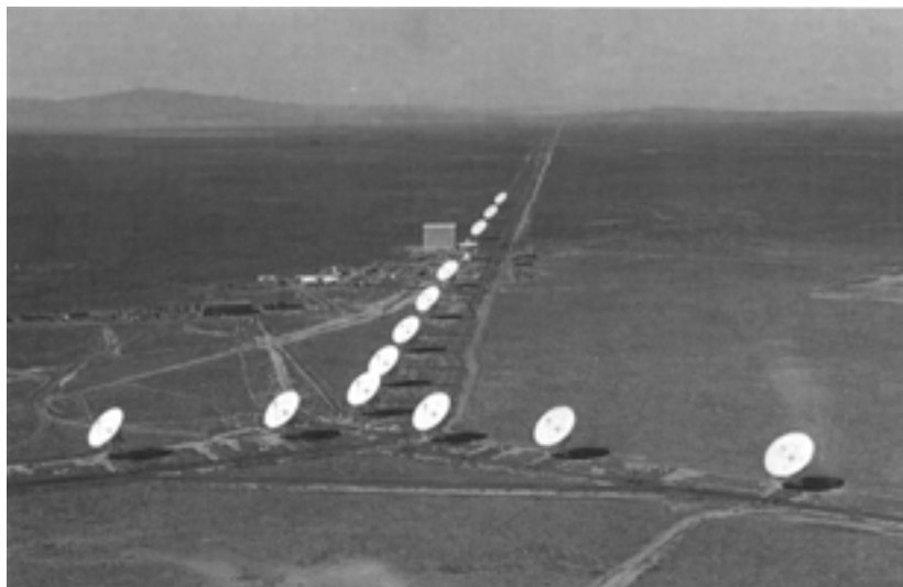
The VLA in the C-configuration, looking down the southwest arm. The sixth telescope along the arm is not in service. Telescope malfunctions occur infrequently and are usually repaired in a few hours. Each of the three arms has nine telescopes. A 28 th was also constructed so that maintenance could be made without interrupting operations of the full array. The spare telescope is housed in the rectangular service building.
