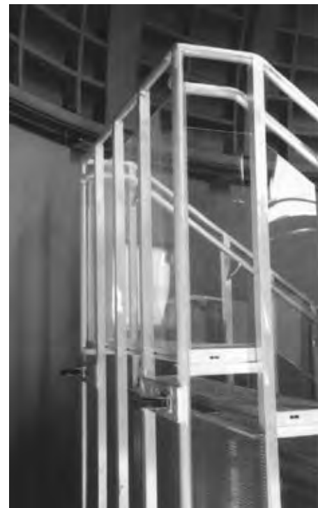
Figure 3 – The back of the observing platform. Note the rear outer wheels, which contact the inner wall of the dome, and the Plexiglas panels installed for safety beneath the handrails.
