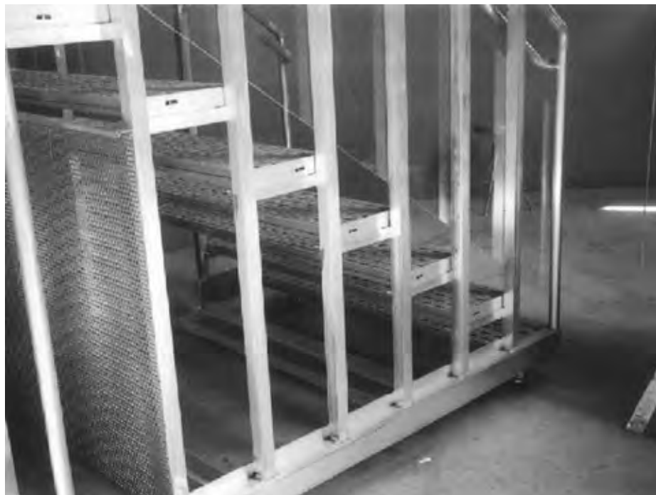
Figure 1 – The full range of motion of the telescope was analyzed and considered in the design of the new platform. Note the large footprint of the observing platform, which is a result of its height.
