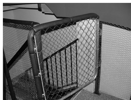
The safety fence and railing.
