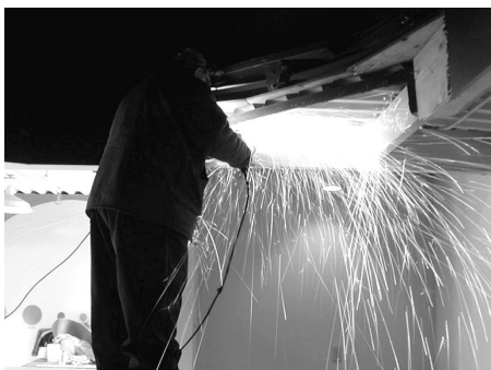
Grinding the frame.
