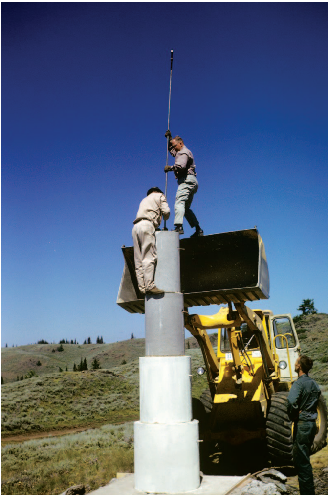
Figure 14 —Snagging the hook seen in Figure 13 with a ring-ended rod that will be used to compress the four concrete cylinders into a rigid pillar to support a solar refractor.
