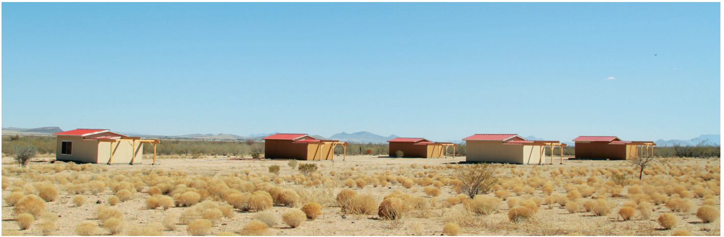
Figure 1 — The standard observatory is 4.5 m (15') square with two piers and a warm room at the roll-off end. These will be ready to use after power and Internet have been connected. The view is to the southeast.
