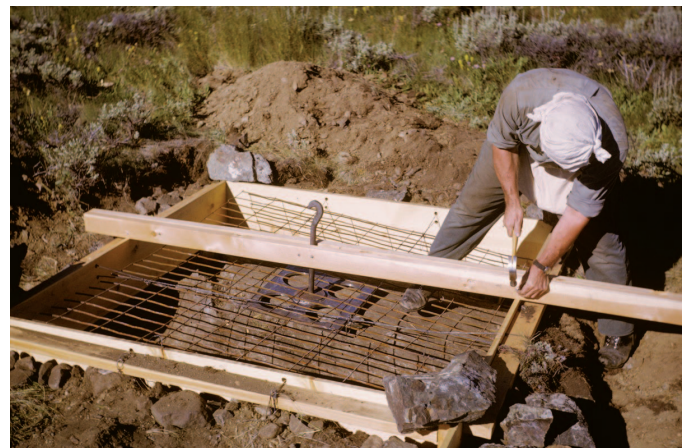
Figure 13 — Mel Lytle builds a form for a cement pad to support a 4-m high concrete pillar for a solar refractor, 1966 July 29.
