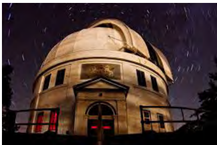
Figure 1 — The Dominion Astrophysical Observatory (1918), in Saanich, outside Victoria, B.C. Its heritage has been preserved, thanks to inspired leadership by Dr. Jim Hesser, by the attached education facility Centre of the Universe, and by strong community support. Source: National Research Council of Canada.
