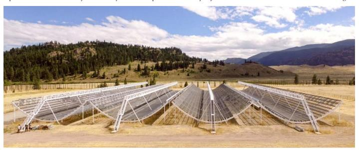
Figure 1 — The CHIME Telescope is designed to provide a large collecting area while also surveying a large part of the sky above the telescope, allowing efficient surveying of the radio sky for FRBs. Image Credit: CHIME
