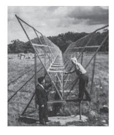
reflector. The sides of the reflector are wire mesh, which acts as a mirror for radio waves. With mirrors 60° to each other, 5 images appear. The real line feed plus its five images act together as an array of long antennas, increasing the sensitivity of the telescope to incoming waves.
